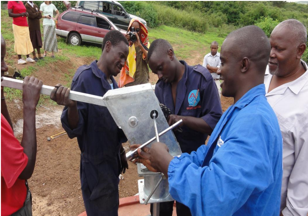
Project in Process
